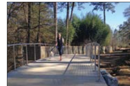
Pictured above is the PermaTrak that was installed on Camp Creek Greenway in 2015.
